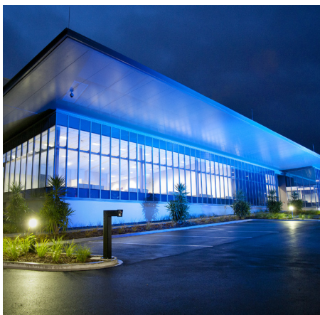
IBM Auckland Data Centre
