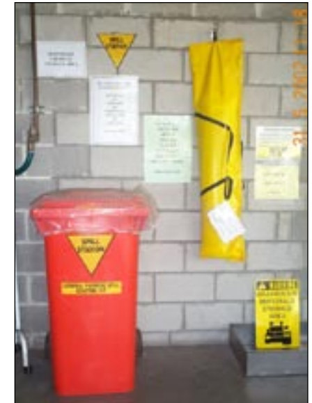
Spill response stations like this one are located as close to the identified environmental hazard as practical
