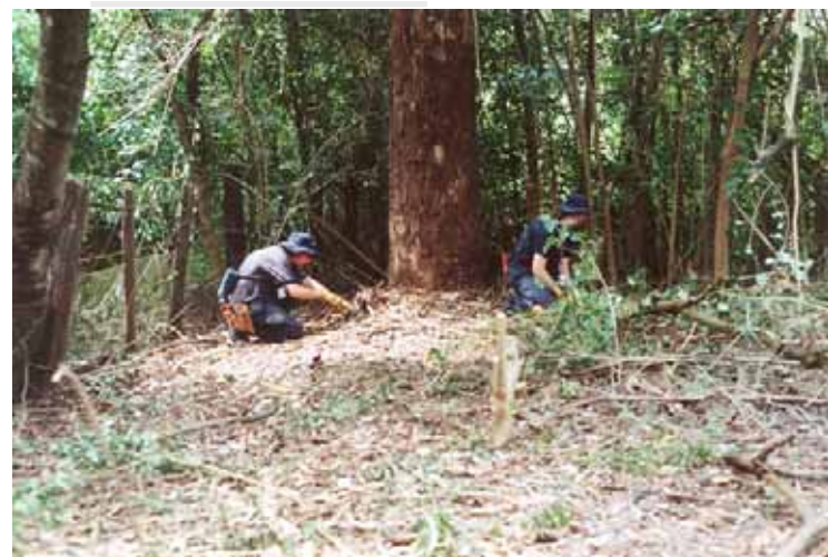
Clearing and weeding of the top area of the West Pennant Hills site
